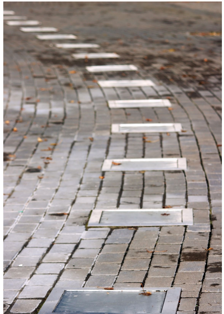
Recessed lighting on walkways and trails can be used to replace more obtrusive overhead lighting. Photo by Shutterstock.
